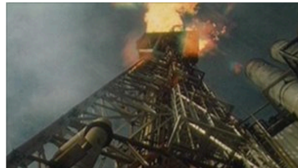
There are about 260 platforms that need to be decommissioned
